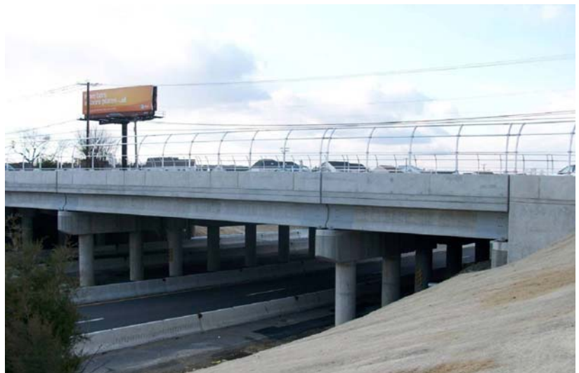
Overview of Bridge No. 37
