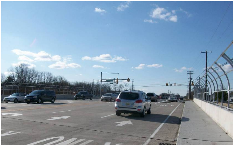
Widening of Bridge No. 37 complete
